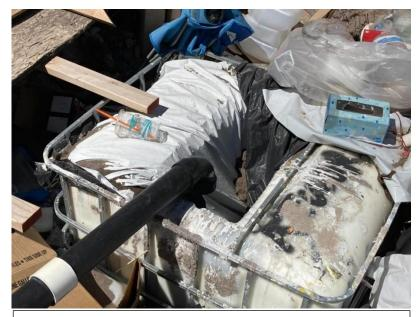
250-gallon caged water container used as an illegal sewage septic system.
