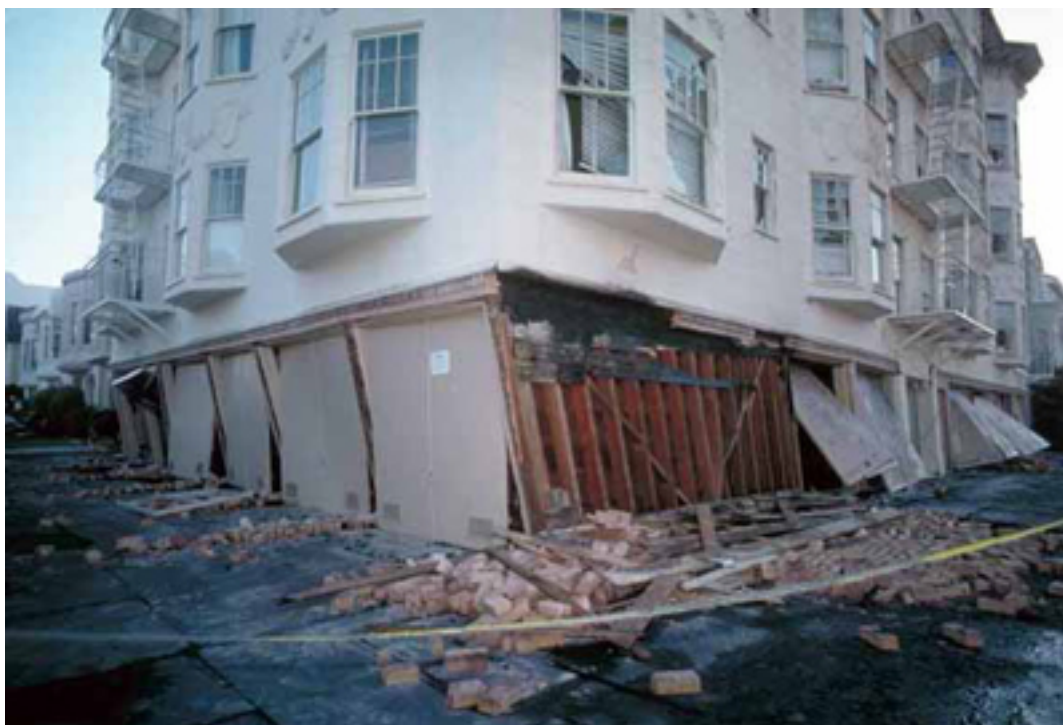
Figure 11-16. Soft-Story Damage from Earthquake
