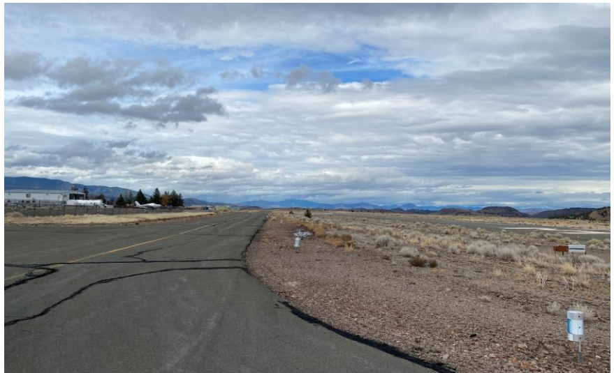
Existing Taxiway - View to the North (Runway on the Right)
