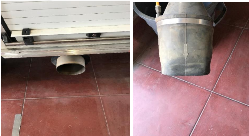
FIGURE 3-6: Vehicle Exhaust System Connectors that are not Compatible with the Assigned Apparatus
