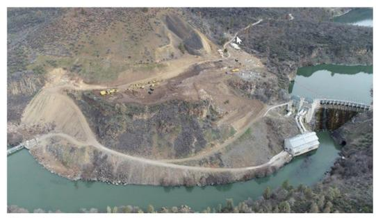
Copco 1 and 2 access roads and waste disposal areas are being established. Existing houses and maintenance building have been demolished. Installed rock fall protection for the powerhouse, penstocks, and access road construction
