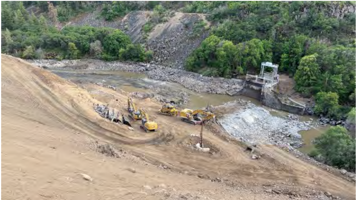
Copco No. 2 dam demolition progress.
