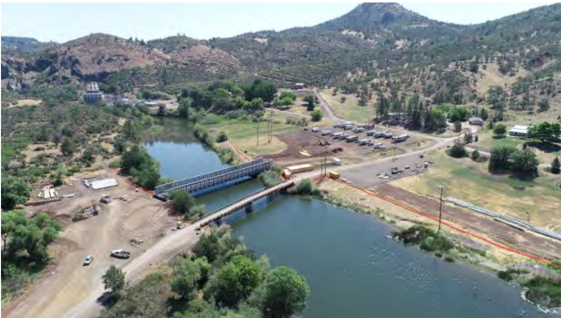
Aerial view showing Copco No. 2 village area and Daggett Bridge.
