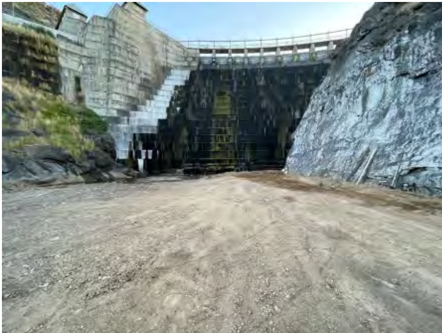
Work pad at the base of Copco No. 1 Dam.
