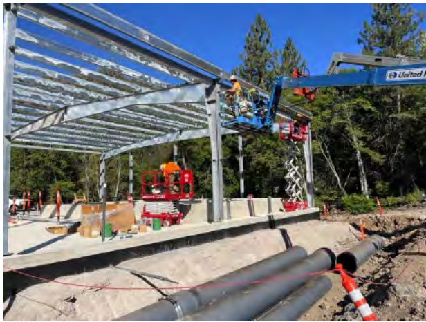
Coho Building – PEMB Erection
