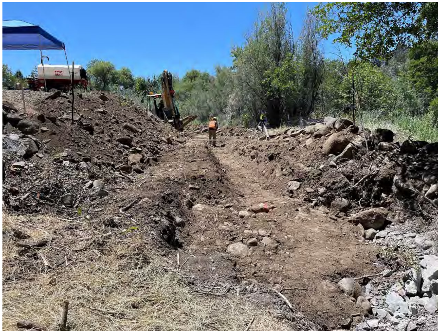
Jenny Creek dry hydrant installation at Copco 2 Village.
