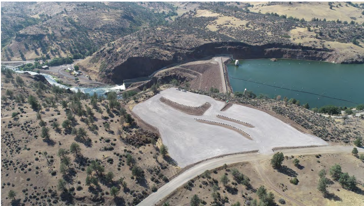
Laydown area on the left abutment at Iron Gate Dam.
