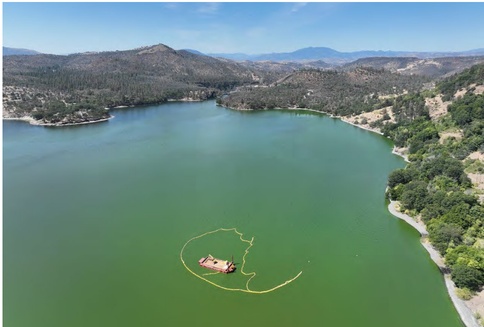
Debris barge in dredging disposal area on Copco Lake.
