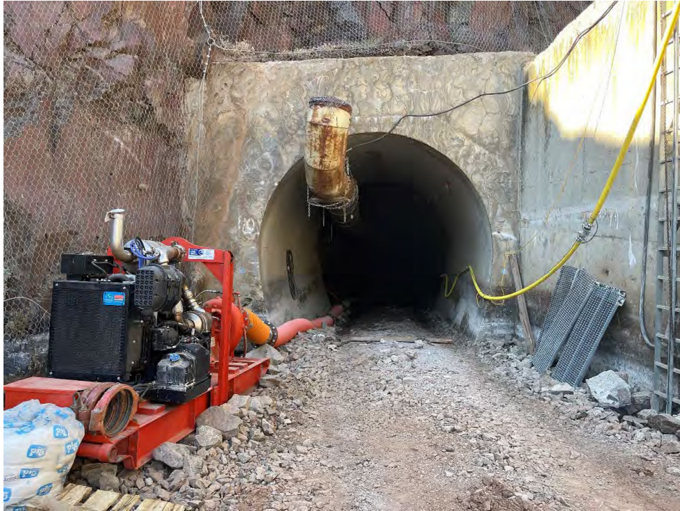
Tunnel portal with temporary vent line at Iron Gate Dam.
