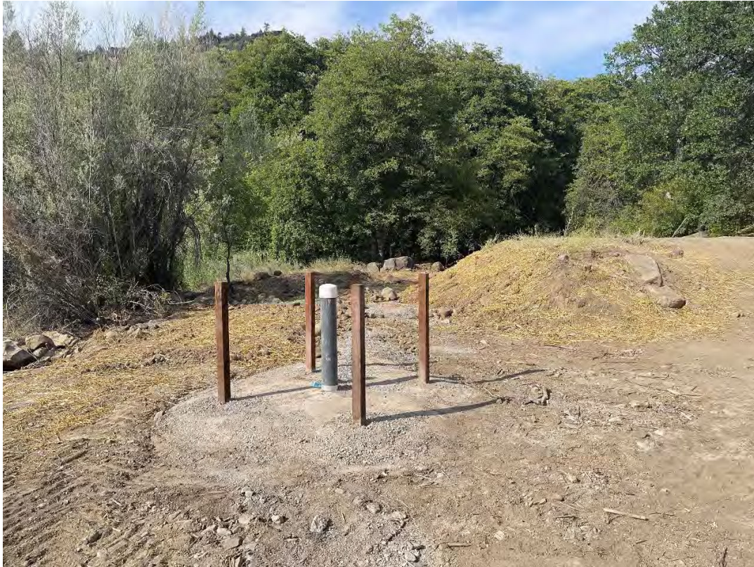
Jenny Creek completed dry hydrant installation at Copco 2 Village.
