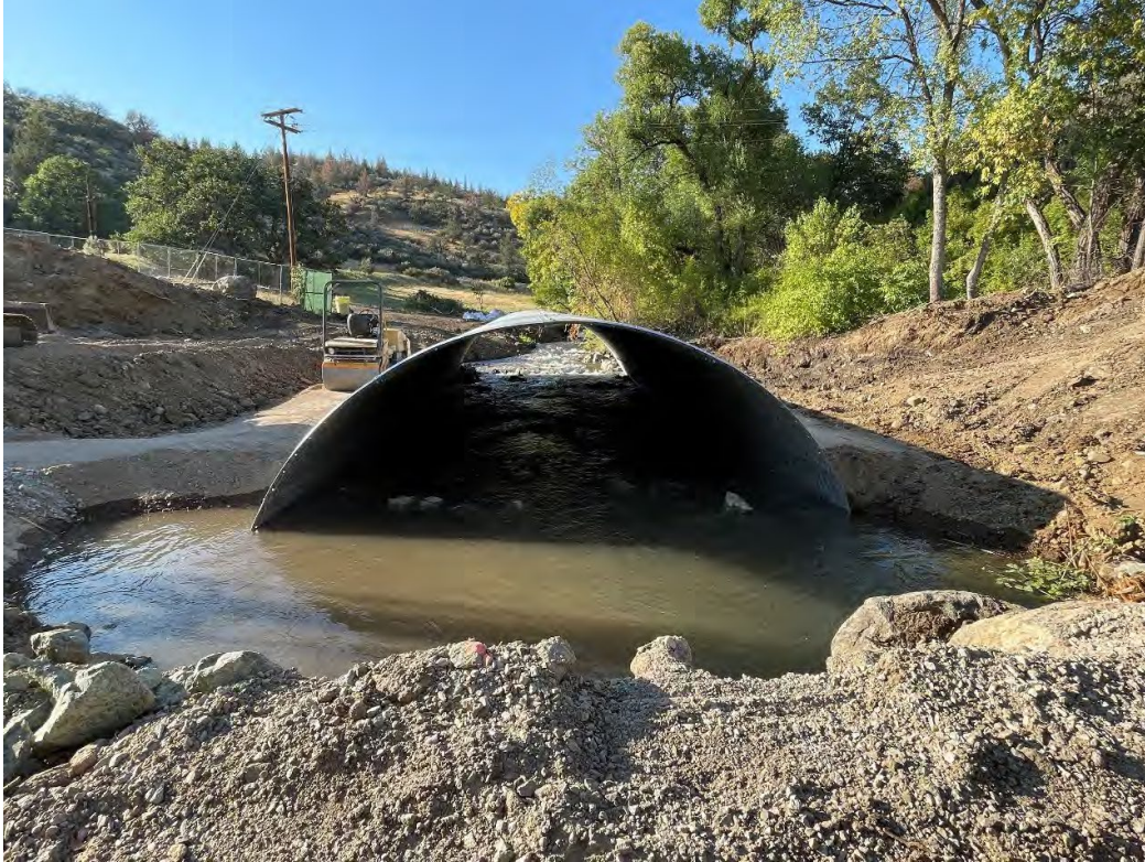
Fall Creek Culvert multiplate arch and backfill at Copco 2 Village.
