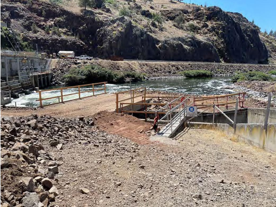
Completed temporary bridge over the fish ladder at Iron Gate Dam.
