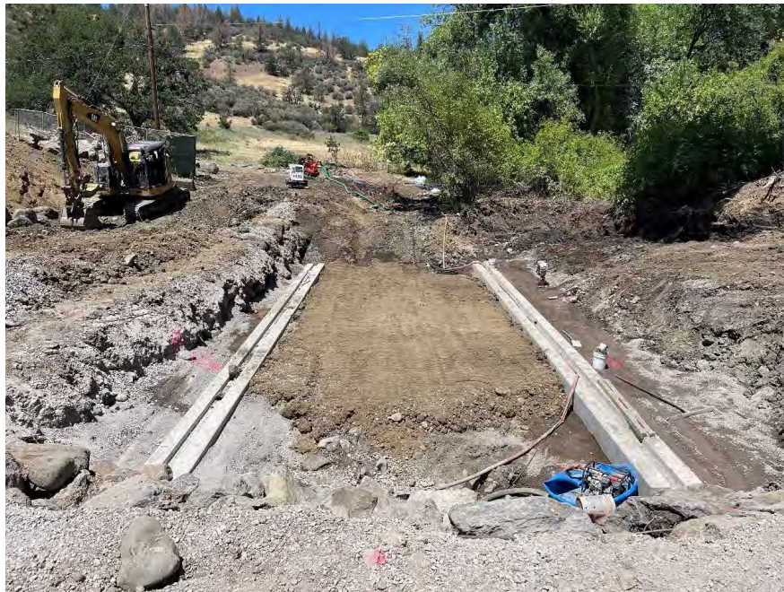
Fall Creek Culvert foundation beams and subgrade at Copco 2 Village.
