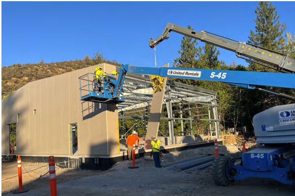
Coho Building – PEMB Wall Panel Install at Fall Creek Hatchery.
