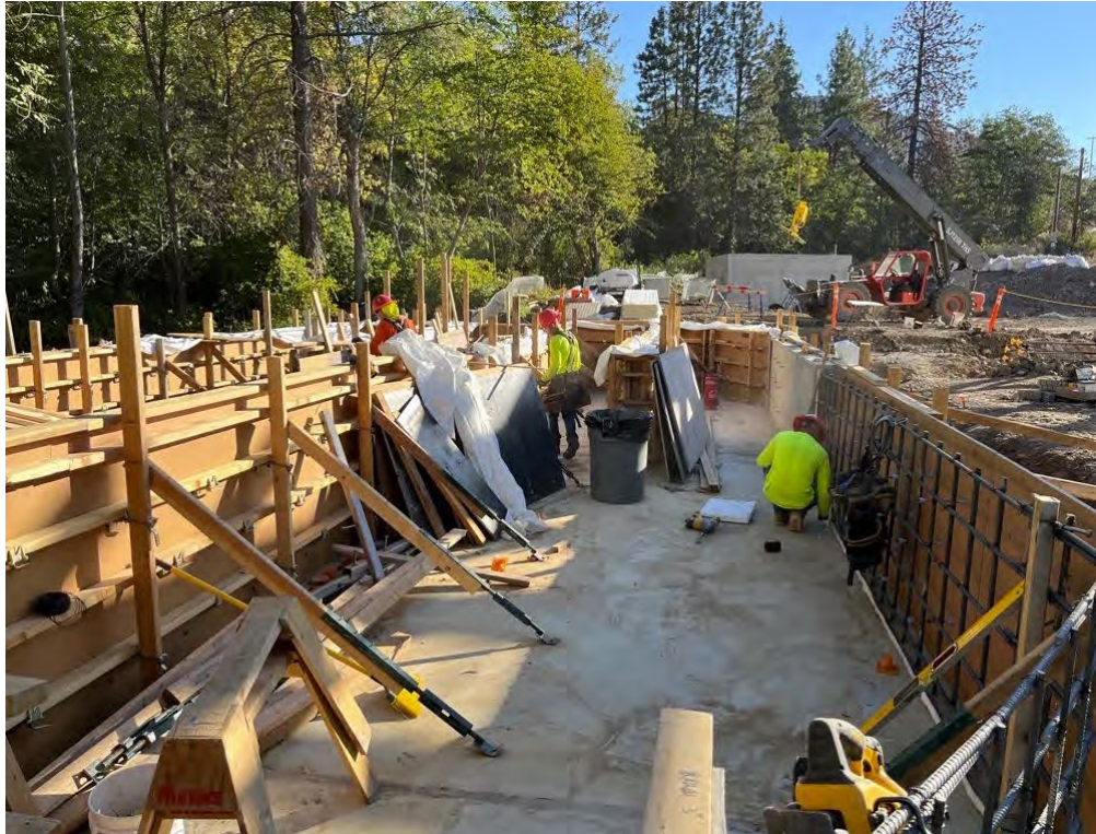
Coho Raceways at Fall Creek Hatchery.
