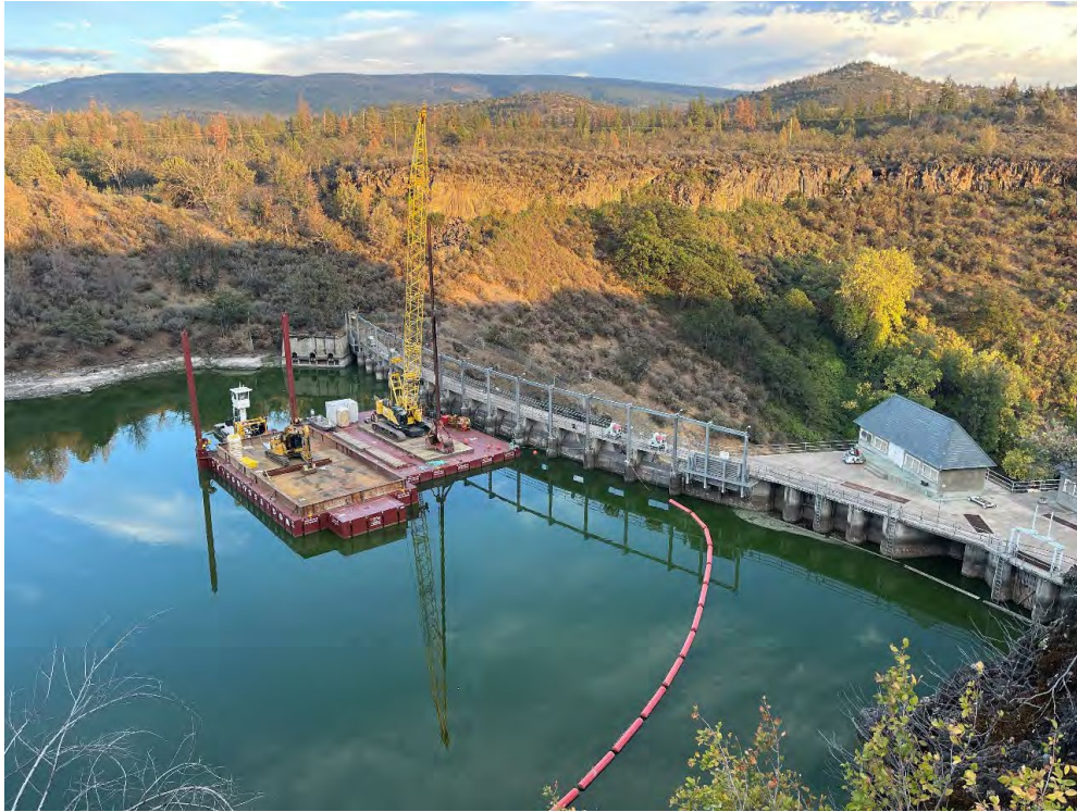
Dredging and debris barges moored at Copco No. 1 Dam.
