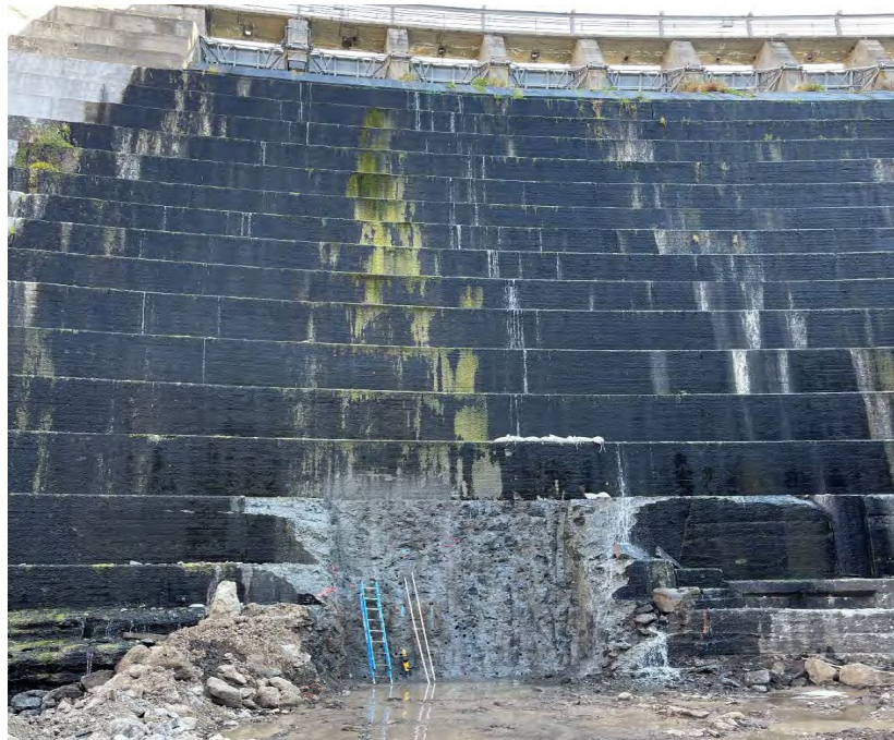
Construction of the Copco No. 1 low-level adit is underway.
