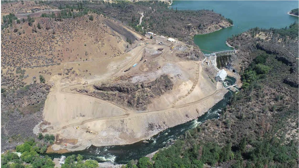
Aerial view showing the overall Copco No. 1 and No. 2 complex.
