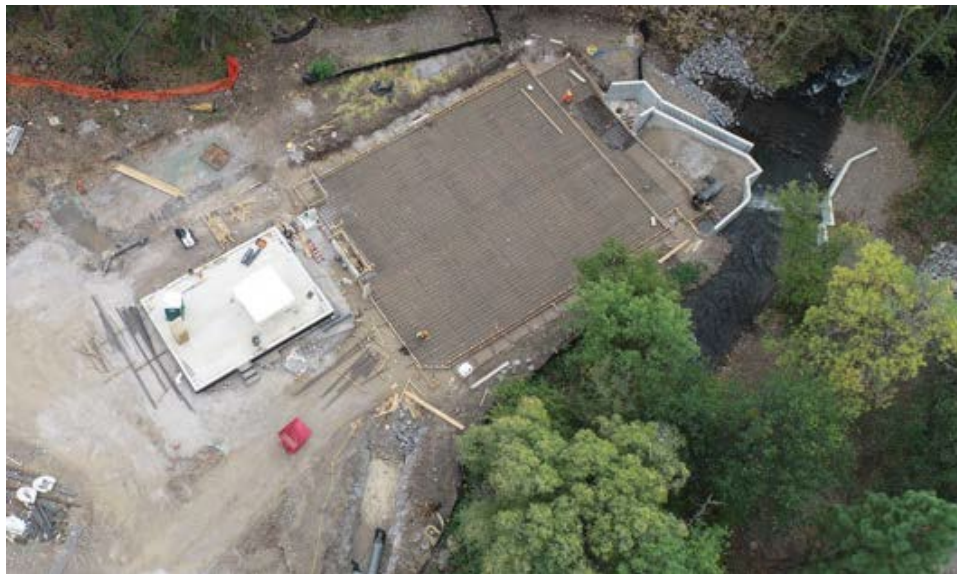
Adult Holding SOG Construction. Fish Ladder and Barrier concrete complete.
