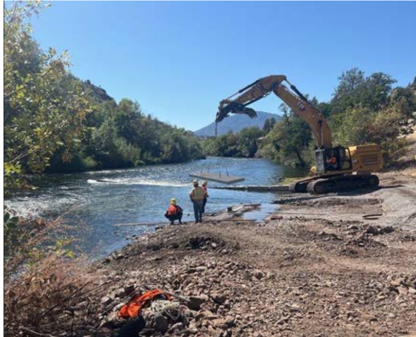
Installing pre-cast concrete panels at the Iron Gate boat ramp
