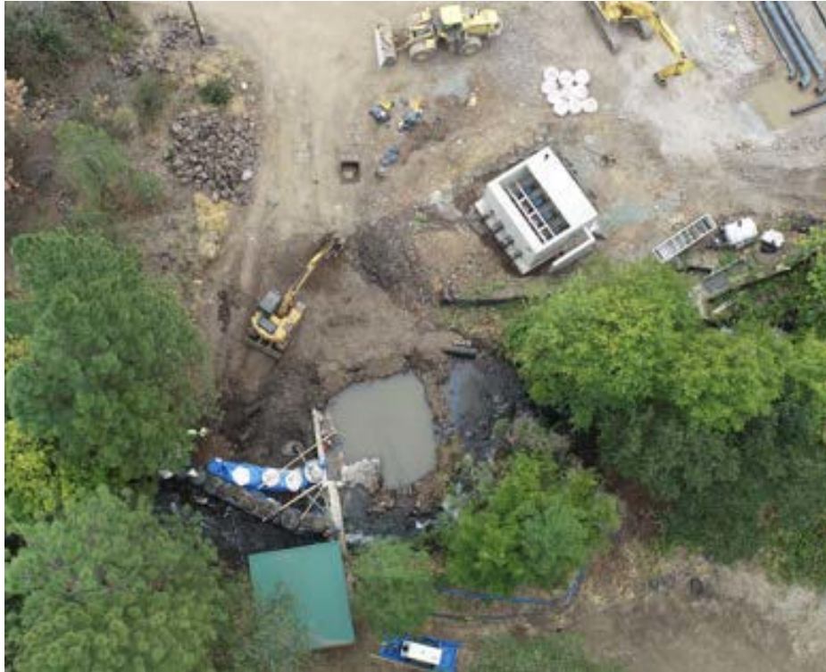
Dam A Construction
