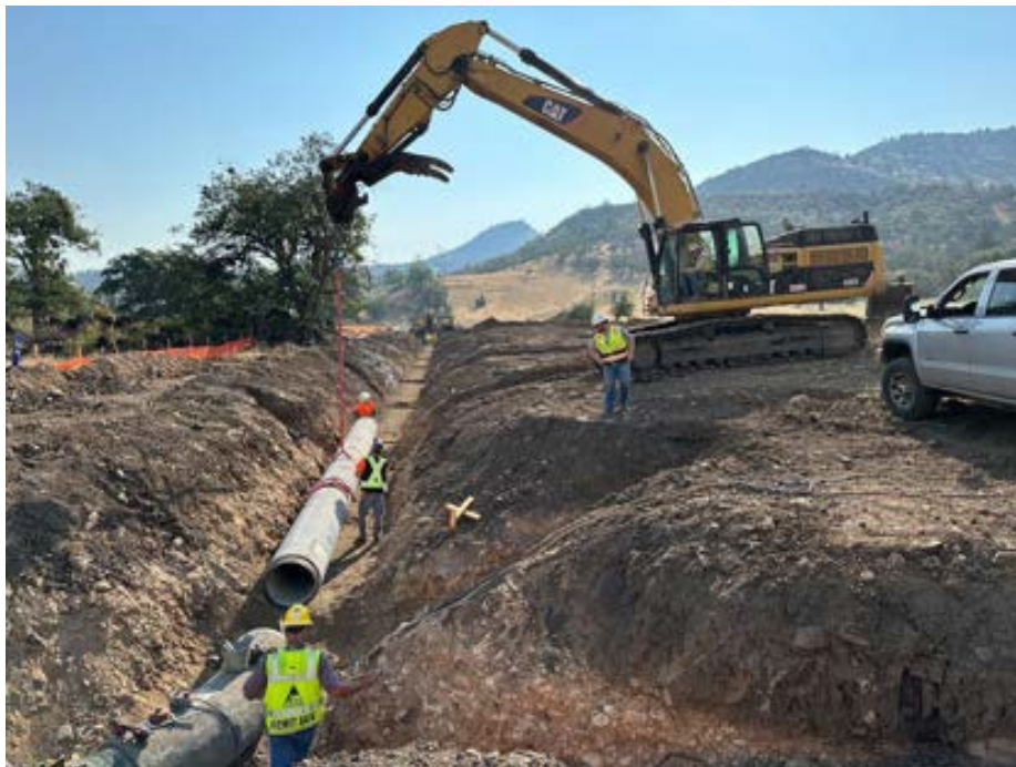
City of Yreka Waterline pipe laying.
