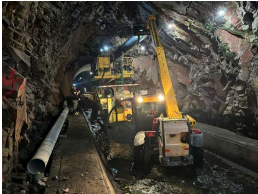
Crew working to hang the new HDPE vent line.
