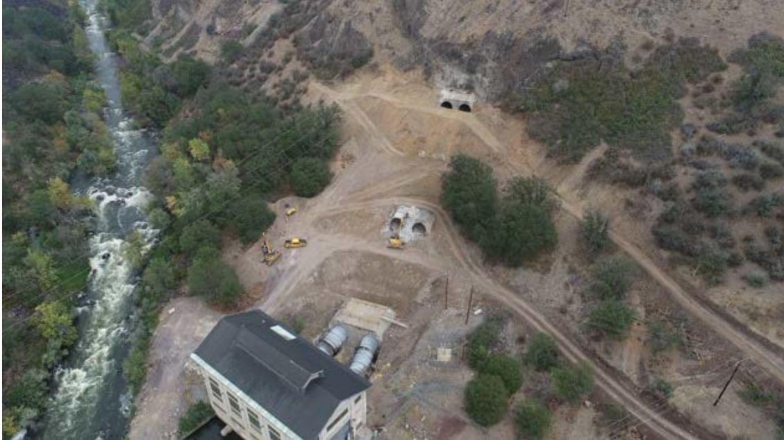
Aerial view showing Copco No. 2 steel penstock demolition progress.
