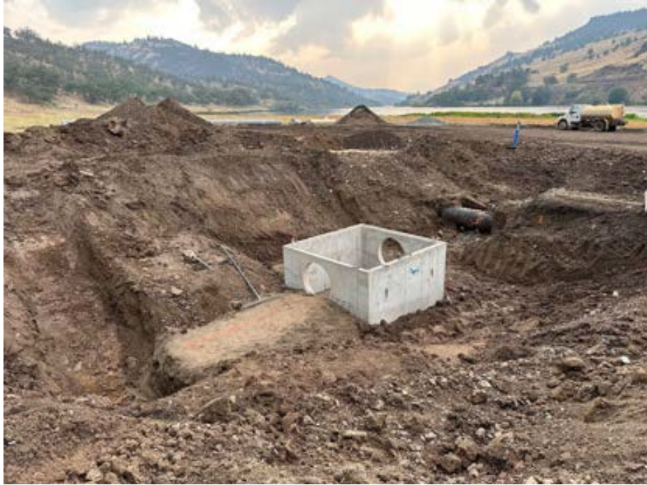
City of Yreka Waterline excavation began at downstream tie-in.
