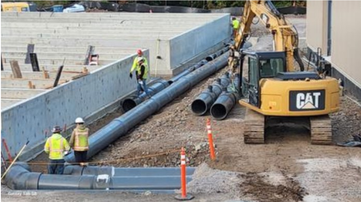
Chinook Raceways & Pipe Install
