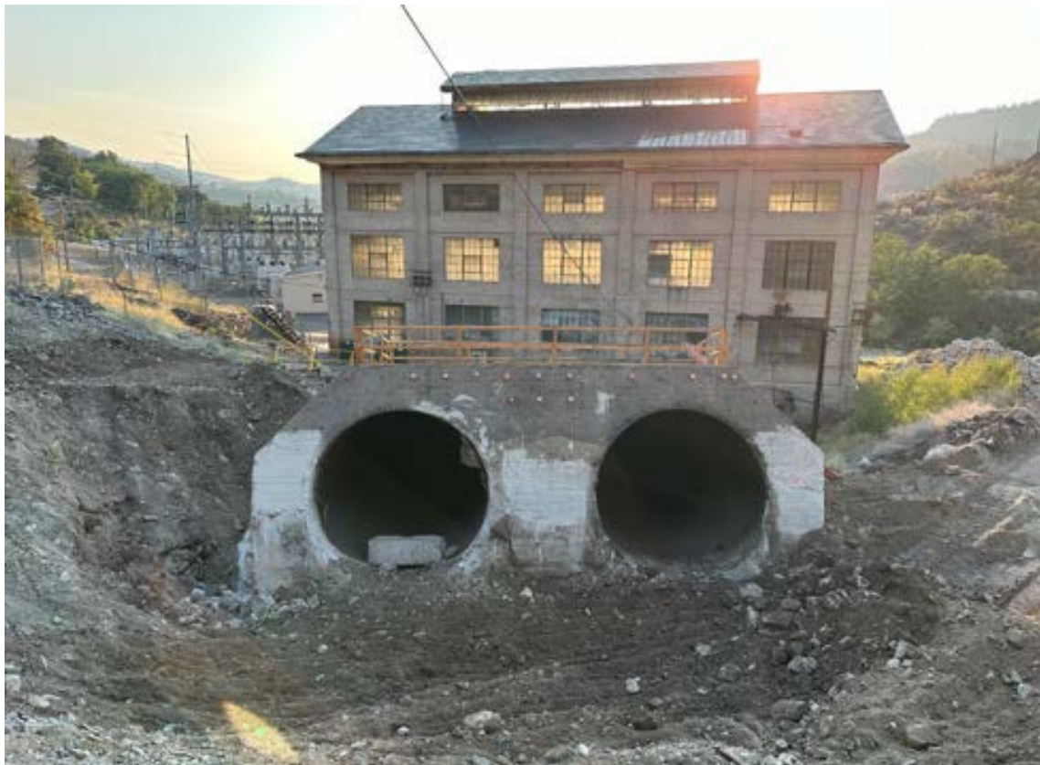
Thrust block at Copco No. 2 that will receive a concrete plug.
