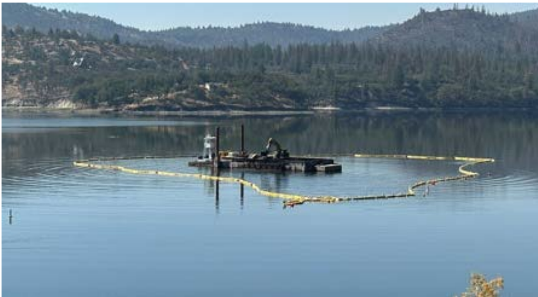
Offloading debris barge in dredging disposal area, Copco Lake.
