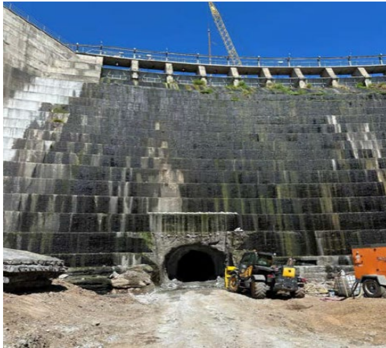
Construction of the Copco No. 1 low-level adit underway.
