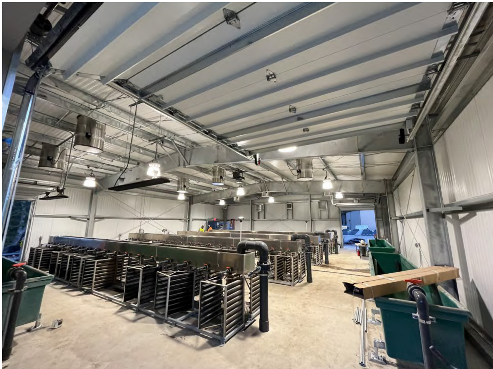
Fall Creek Hatchery progress. Chinook Incubation Building.
