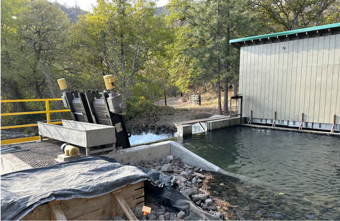
Dam A Velocity Barrier & Hatchery Intake
