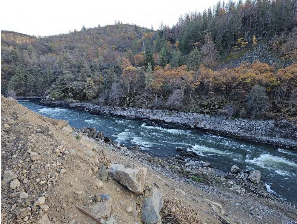
Klamath River channel downstream from Copco No. 1 powerhouse.
