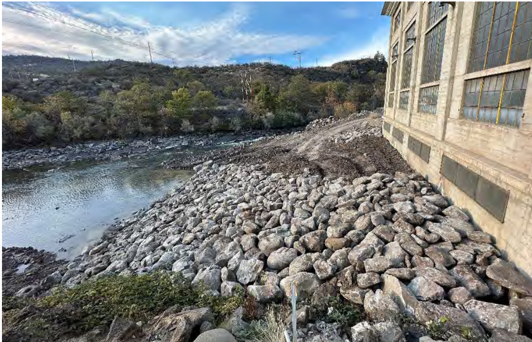
Copco 2 tailrace backfill progress – rip rap partially completed.
