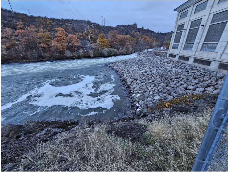
Copco 2 tailrace backfill progress – rip rap completed.
