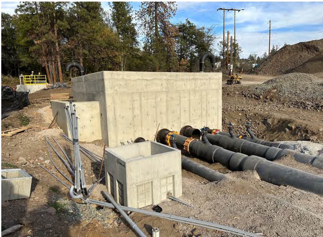
Pipe Installation: Downstream of Meter Vault
