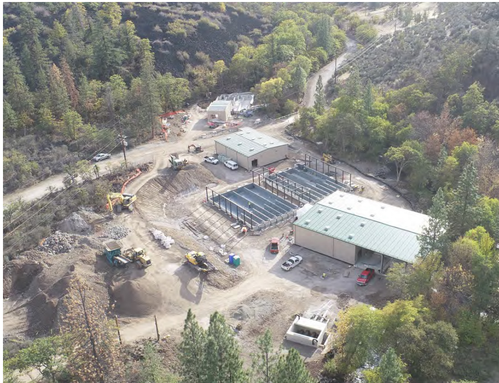
Overview of Fall Creek Hatchery progress.
