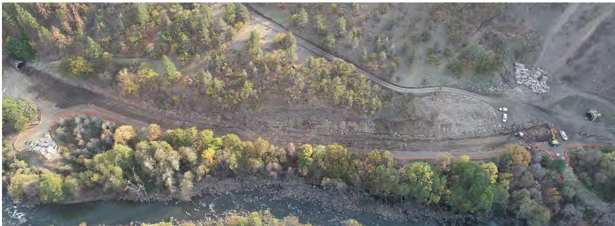
Copco 2 wood stave flowline soil remediation progress.
