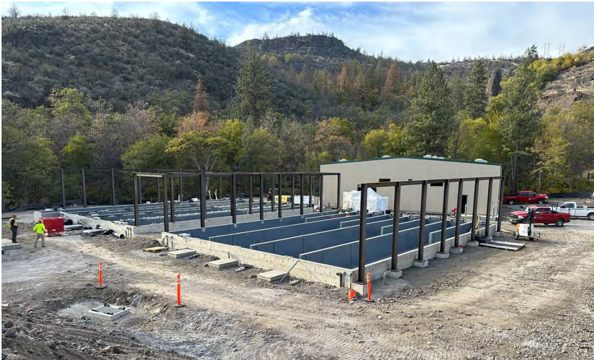
Chinook Raceways & Bird Netting Install
