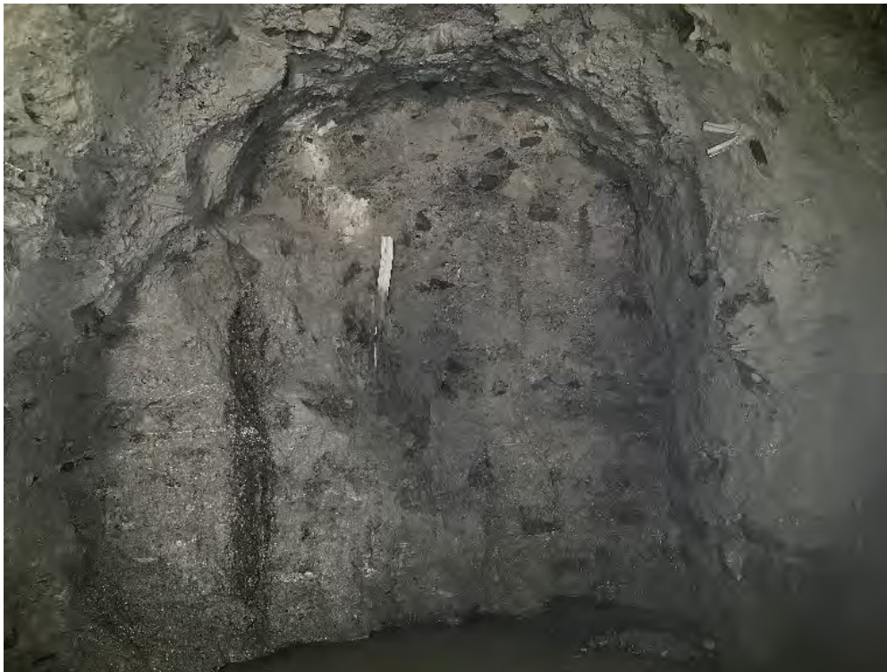
Face of the plug round after the last blast in the Copco 1 adit at Copco 1.
