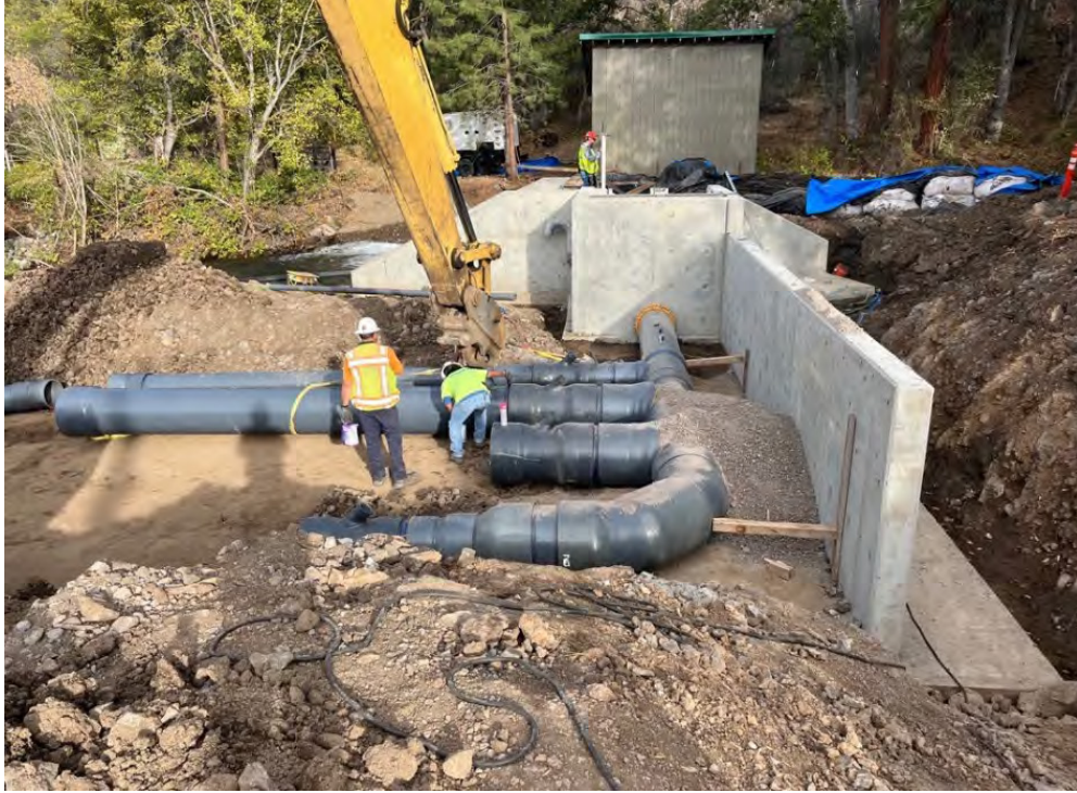
Dam A velocity barrier and intake construction.
