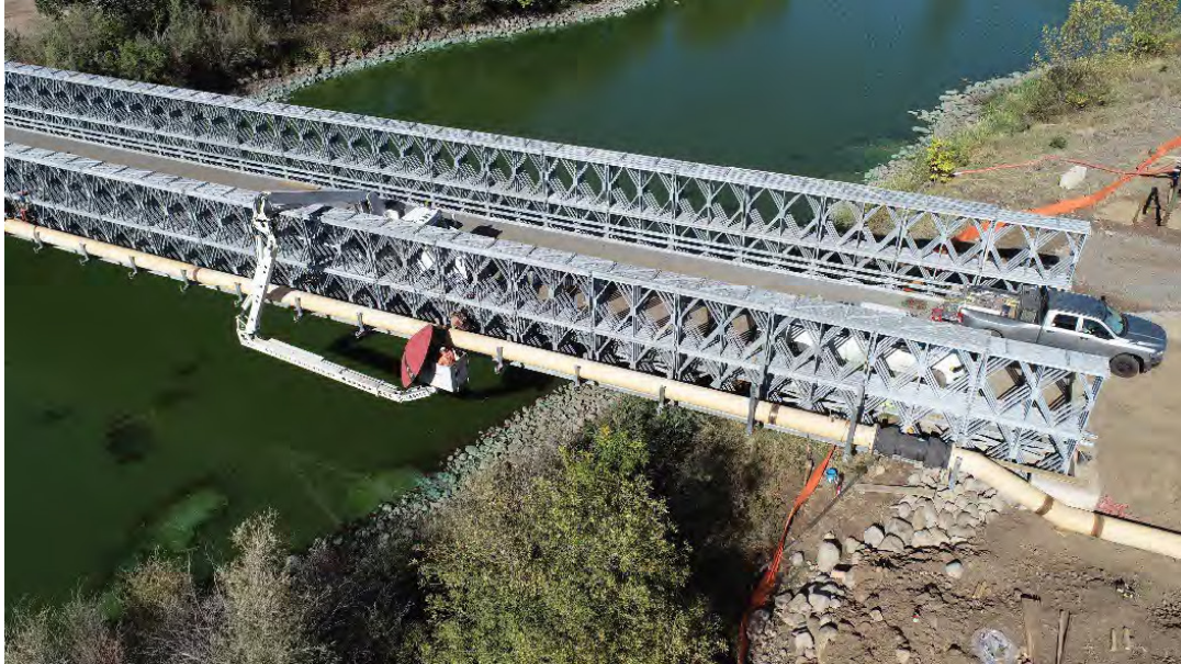
Welding pipe across the new Daggett Bridge from a snooper truck.
