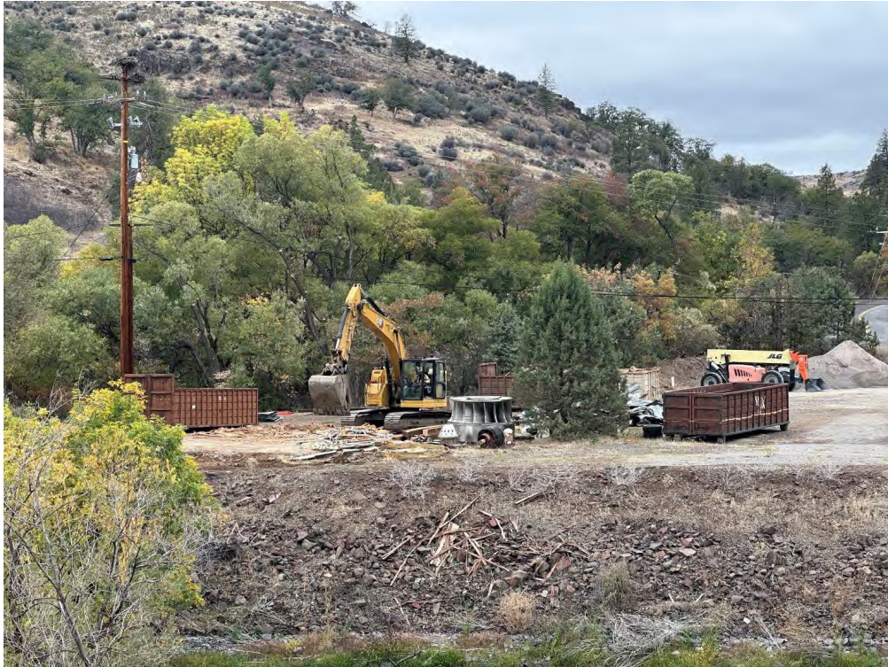
Demolishing storage shed near Iron Gate operator houses.
