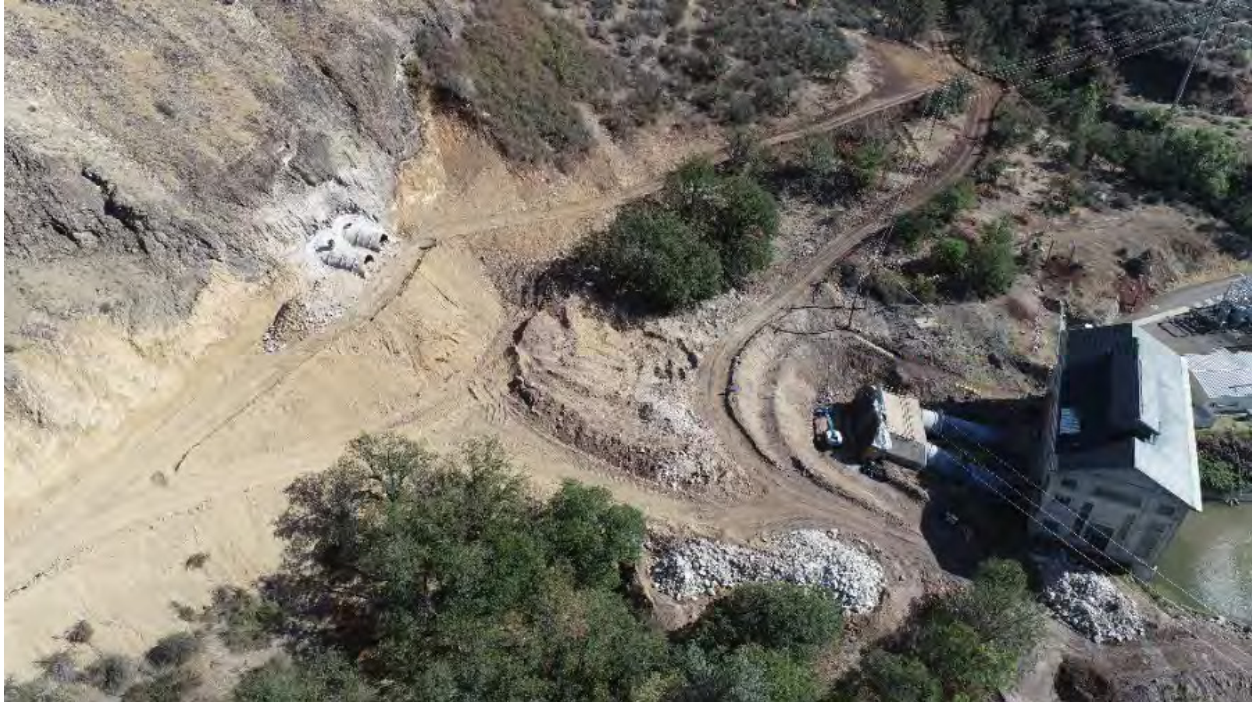
Copco 2 steel penstock thrust blocks have been removed.
