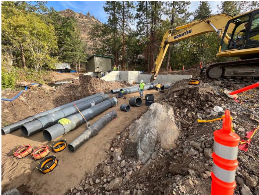
Pipe installation: Intake to meter vault.
