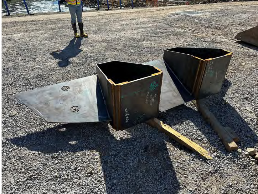
Steel wrapper from the super-cavitating baffles, viewed from the upstream side.
