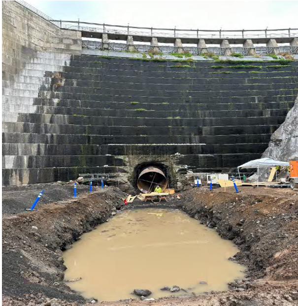
First steel extension pipe segment and excavated trench for the second and third segments at Copco 1 adit tunnel.
