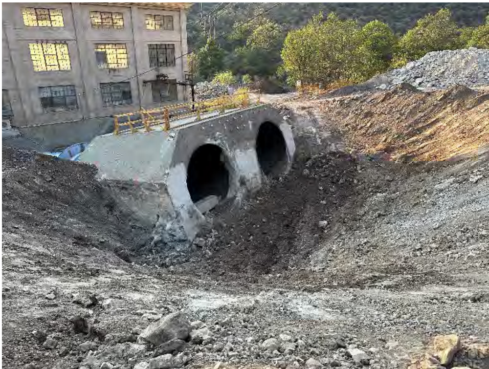
Copco 2 lower thrust block exposed in preparation for permanent concrete plug.
