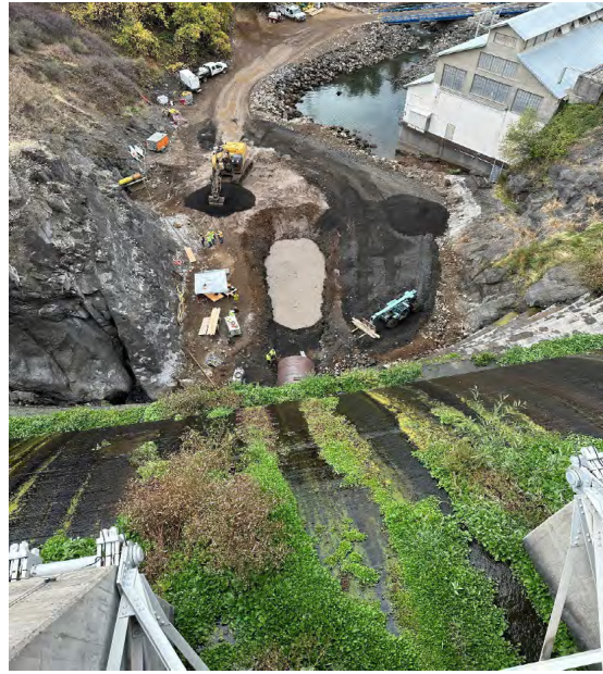
First steel extension pipe segment and excavated trench for the second and third segments at Copco 1 adit tunnel.
