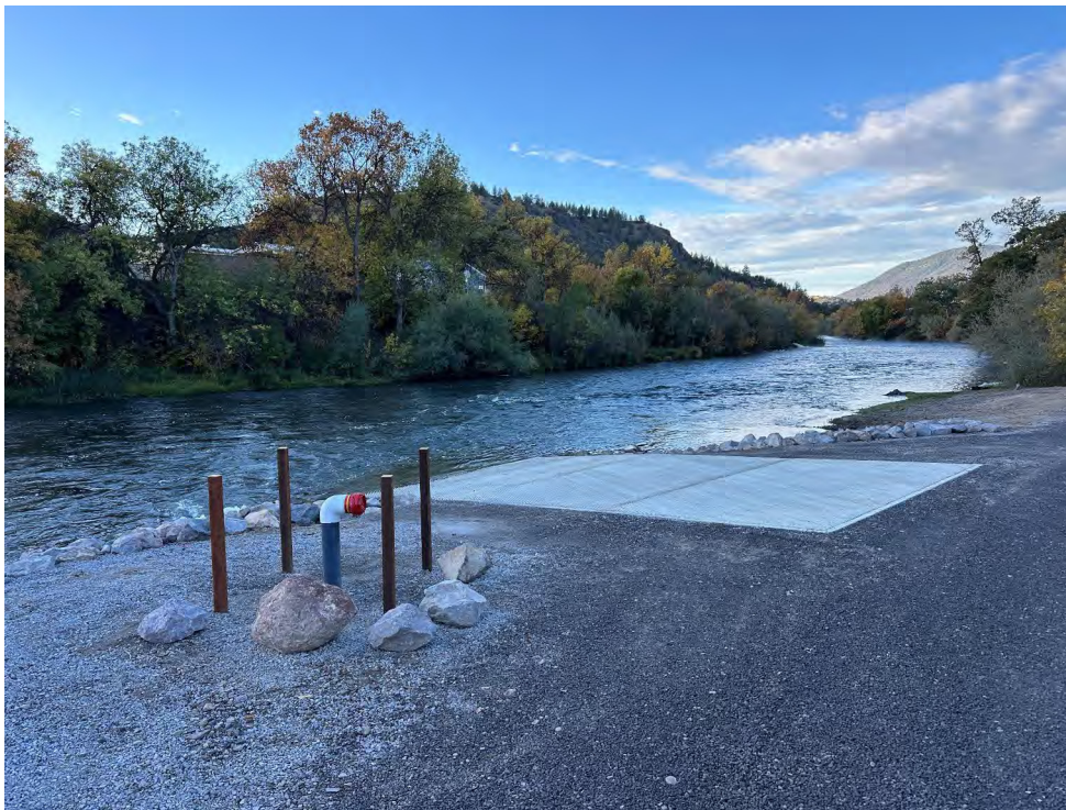
Completed Iron Gate boat ramp and dry hydrant.
