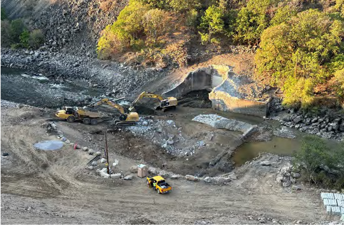
Loading out concrete rubble from first blast at Copco 2 foundation.
