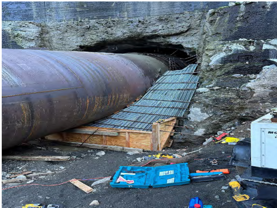
Copco 1 – framework in place for steel extension pipe.
