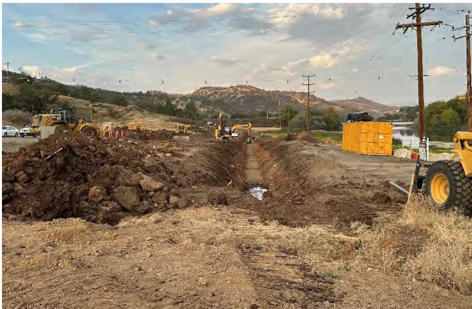
City of Yreka waterline excavation approach the new Daggett Bridge.
