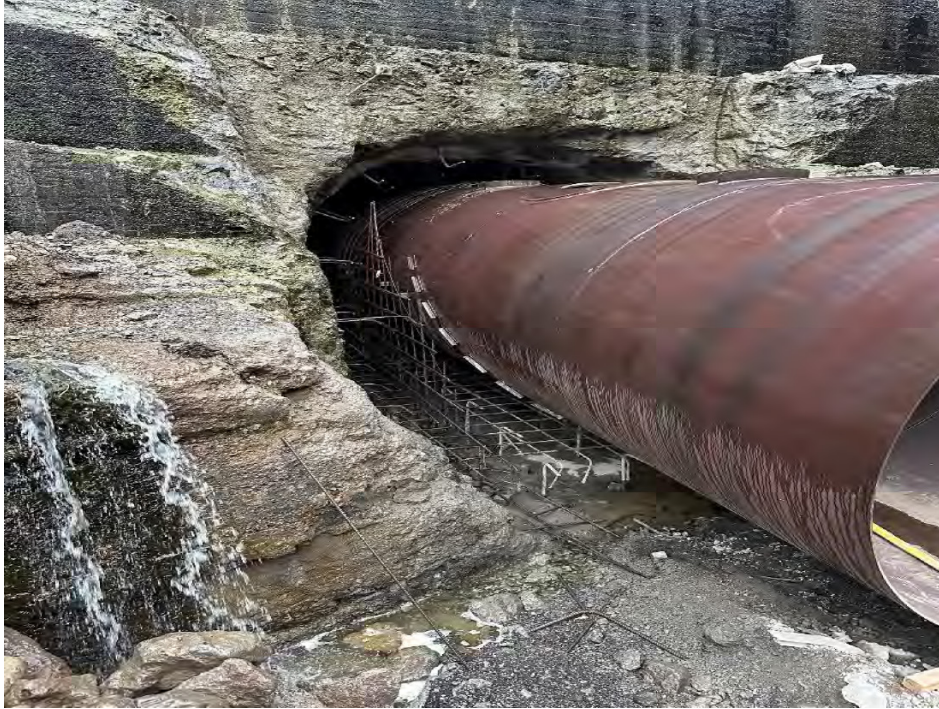
Steel extension pipe set in place with rebar at Copco 1.
