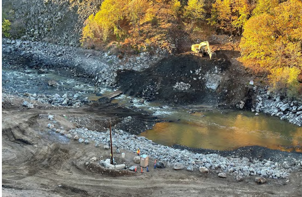
Grading over the former Copco 2 intake structure.
