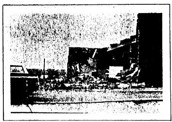
Even reinforced masonry failed similarly to tilt-up walls in the 1971 San Fernando earthquake in the industrial buildings.
