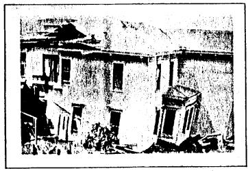
House built across fault at Wright's Station. 1906 earthquake.
